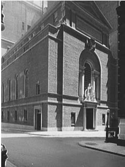
Church of Our Lady of Victory 60 William Street NY, NY 10005
